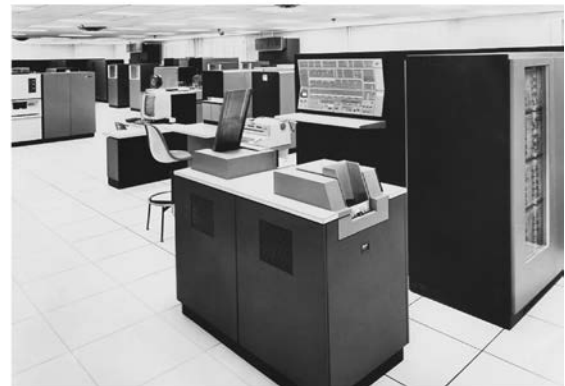
FIGURE e1.13.3 IBM System/360 computers: models 40, 50, 65, and 75 were all introduced in 1964. These four models varied in cost and performance by a factor of almost 10; it grows to 25 if we include models 20 and 30 (not shown). The clock rate, range of memory sizes, and approximate price for only the processor and memory of average size: (a) model 40, 1.6 MHz, 32 KB–256 KB, $225,000; (b) model 50, 2.0 MHz, 128 KB–256 KB, $550,000; (c) model 65, 5.0 MHz, 256 KB–1 MB, $1,200,000; and (d) model 75, 5.1 MHz, 256 KB–1 MB, $1,900,000. Adding I/O devices typically increased the price by factors of 1.8 to 3.5, with higher factors for cheaper models.
