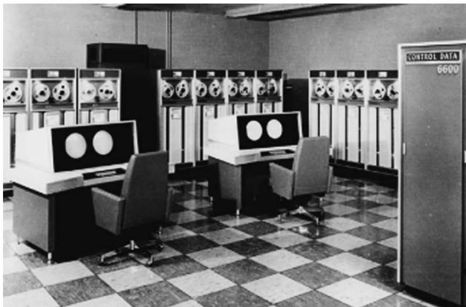
FIGURE e4.17.2 The CDC 6600, the first supercomputer.
